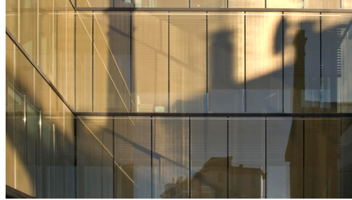
C Quadro, Executive Building, Udine, IT
