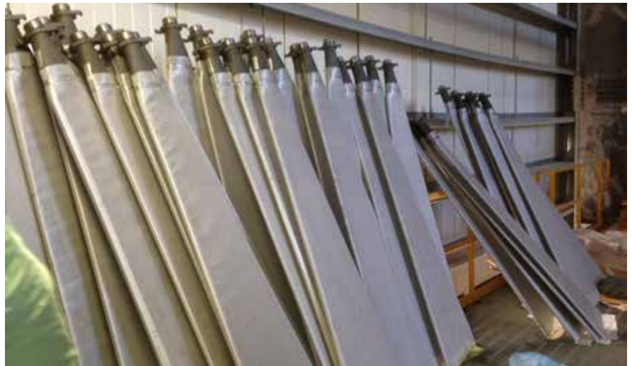
Filter segments ready for installation
